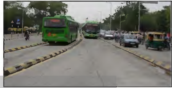
Figure 15: Only kerbs used in Delhi to segregate bus lane from main carriageway
